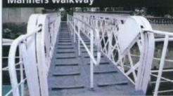
Coat 1: Jotamastic 87 (Epoxy mastic) + 10% Thinners @150 microns dft Coat 2: Jota Armour AS @ 1000 microns dft
