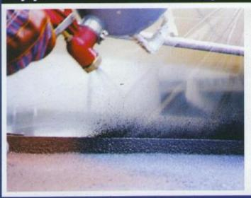
Jota Armour has been specially formulated to enable application by the simplest of methods. There is no requirement for expensive application equipment or the need for extensive experience to apply this product. All you need to apply Jota Armour AS is a small air compressor (circa 3.5 bar), air hose and a Gravity Feed Hopper Gun for larger areas or stipple brush for smaller areas, keeping application costs to the minimum.
